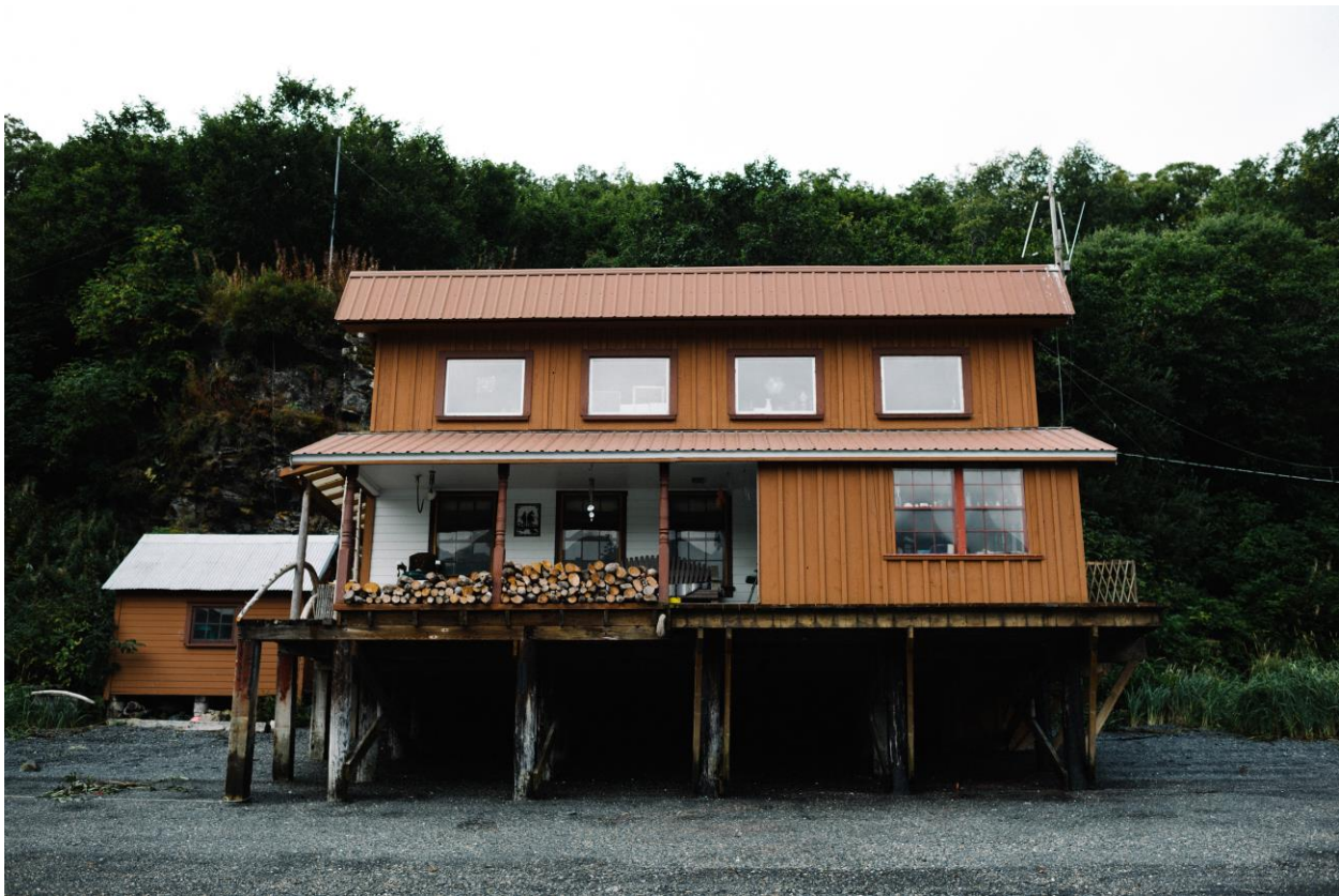
Pilings under the house. P-1000-8-104.
